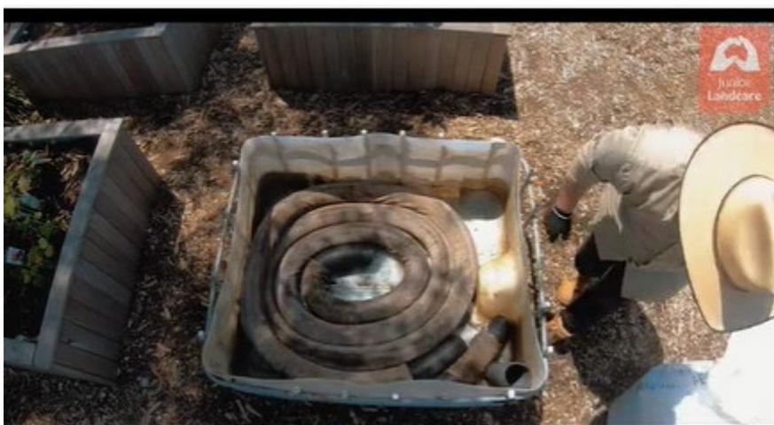
Step number 3: Add some gravel around and the pipe. The gravel is used to fill the gaps around the pipe so that the soil layer can sit nice and evenly on the top of the pipe and get wet. You will need to use scoria, less than 7mm or ¼ minus gravel for effective capillary action.
